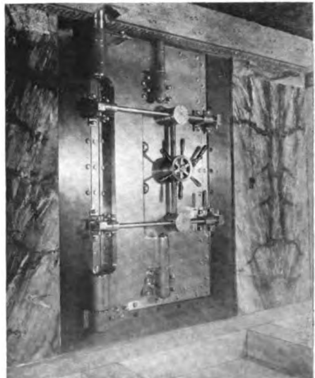
VAULT DOOR CLOSED
